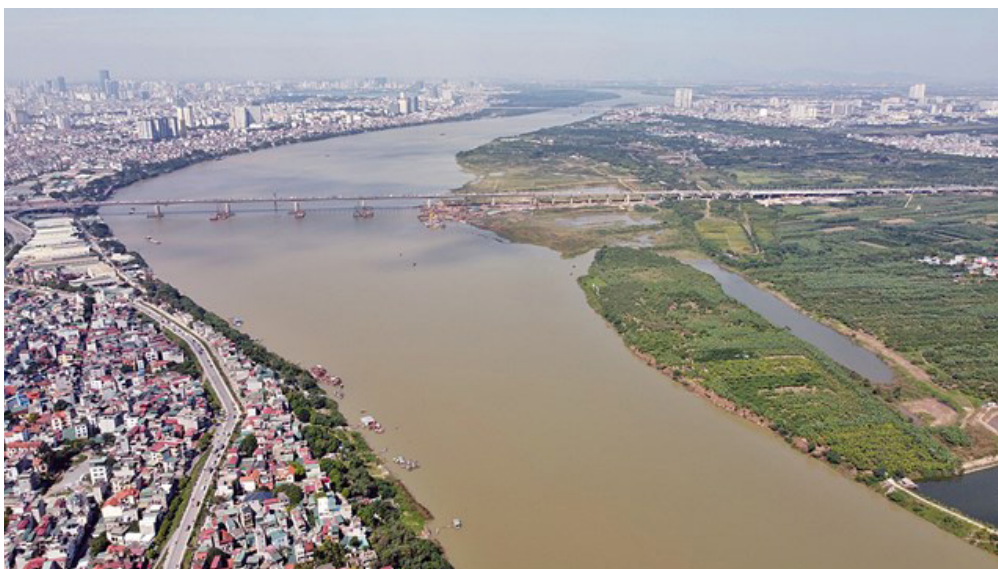
▲ A section of the Red river flowing through Ha Noi City
